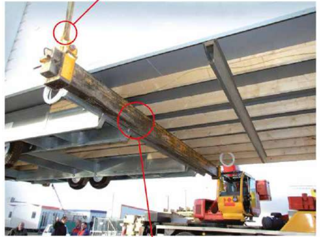
Perpendicular lifting bar with cross member and near to the central metal part.
