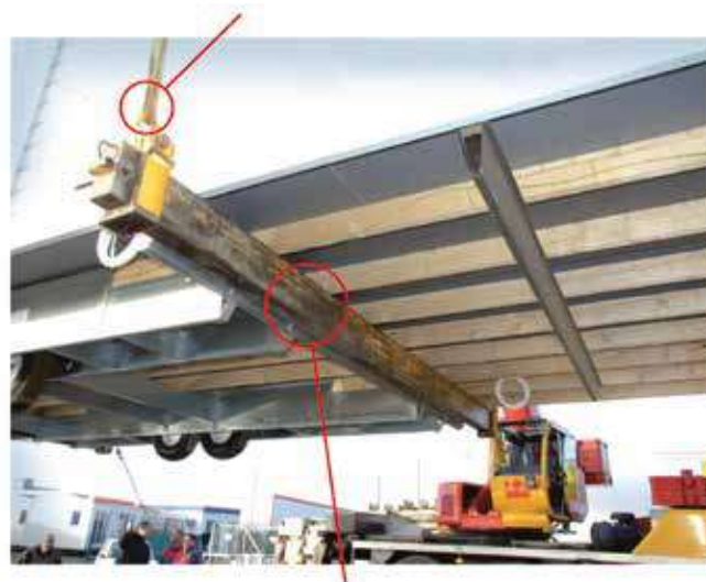
Perpendicular lifting bar with cross member and near to the central metal part.
