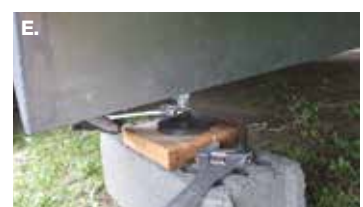
Finish adjustment by using the jacks and an adjustable spanner.
