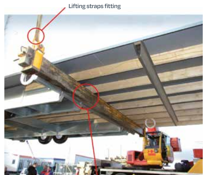
Perpendicular lifting bar with cross member and near to the central metal part.
