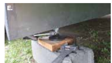
Finish adjustment by using the jacks and an adjustable spanner.
